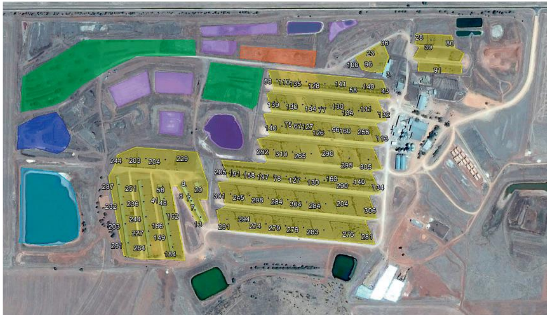
The feedlot layout : 17 431 cattle. Features of the feedlot are: cattle pens (yellow); manure stockpiles (green); effluent pools (purple); mortality composting (dark blue); main water storage (light blue); and sediment pond (orange)_Hacker et al. 2016
