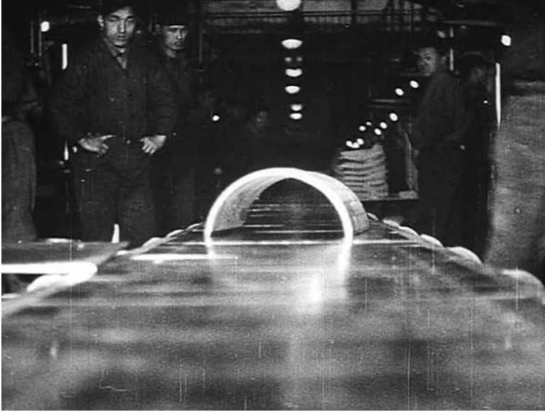
FIGURE 6.7 A plate on the conveyer belt, The “Morning Sun” Shines.
