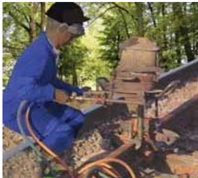
Figure 3.11 Thermit process for joining railway tracks
